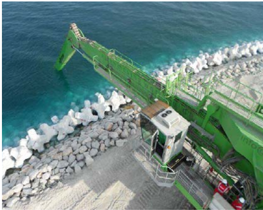
Figure 34: Custom made balance crane with camera and echographic image recognition
