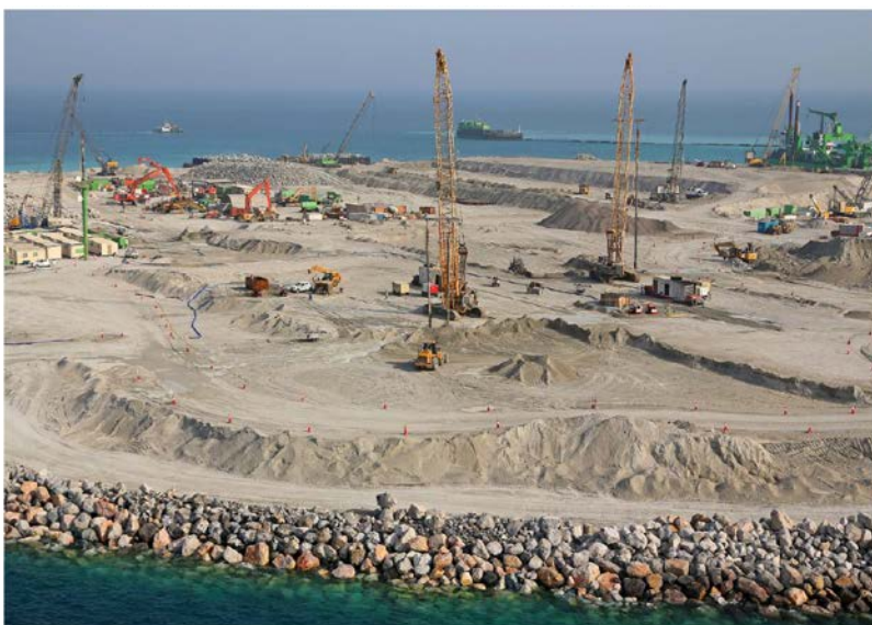
Figure 35: Multitude of activities, incl. vibro compaction
