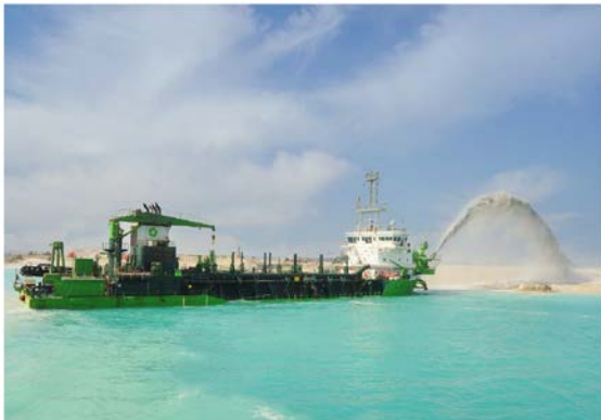
Figure 31 Sand fill by TSHD
