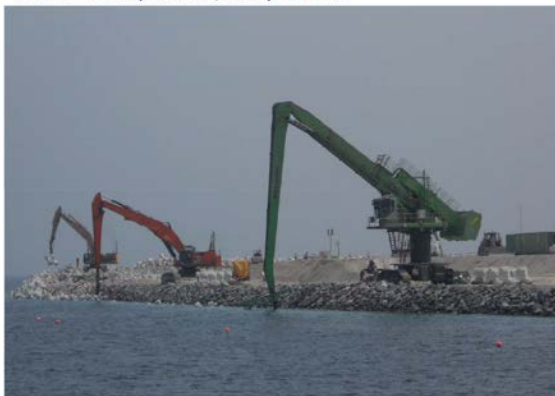
Figure 32 Shore protection installation (Accropodes train)
