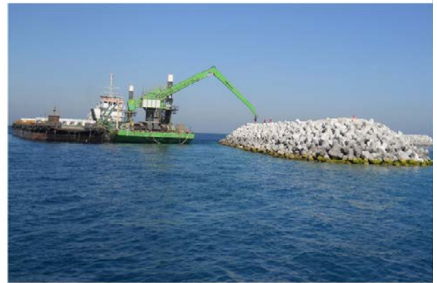
Figure 34: Custom made balance crane with camera and echographic image recognition
